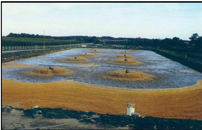
Typical Large TYPHOON Aerator Lagoon Installation
