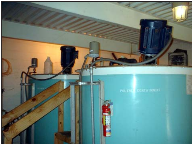
Typical RIPTIDE Mixer in a tank.
