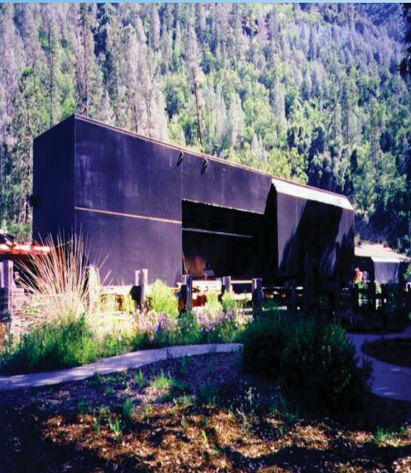
Prefabricated Wastewater Package Plant, Leadville, CO.
